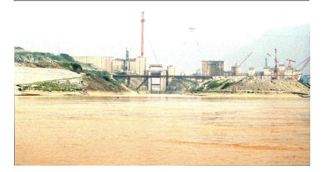
The Three Gorges Dam project, the largest of its kind anywhere in the world, is to be located near Yichang in Hubei Province. The scheme is China's largest multi-purpose project generating electricity, improving flood control and navigation and providing water. The crest of the Dam will be nearly 2000m long and 185m high. A 595km long reservoir will be created and the turbines will generate 18.2Gw (giga watts) of energy - enough to supply the current needs of most of central and eastern China.
